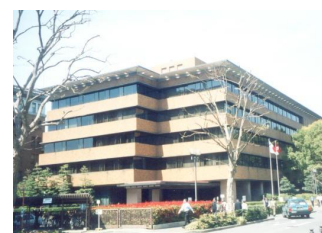
Assembly Building September 1975
